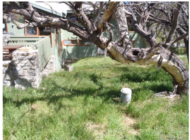
Figure 14: Photo of the underground electricity adjacent to the lodge
