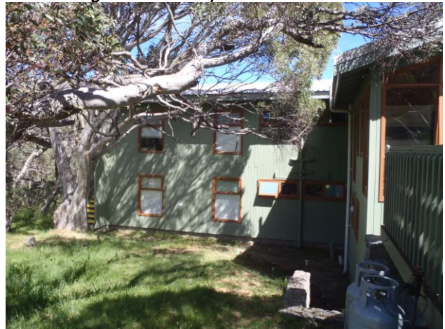
Figure 8: Photo of the eastern side of the lodge
