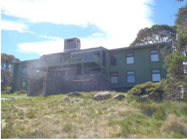
Figure 3: Photo of the western side of the lodge from the Link Road
